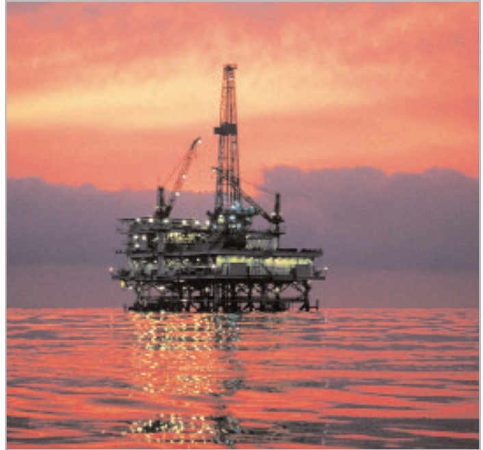
Isolated and hazardous locations are often ideal candidates for remote monitoring and diagnostics programs.
