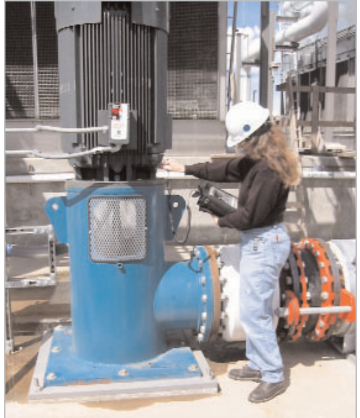
In some applications where in-house resources or expertise is limited, machine condition data can be collected manually and then sent to a central location or a third party for analysis.
